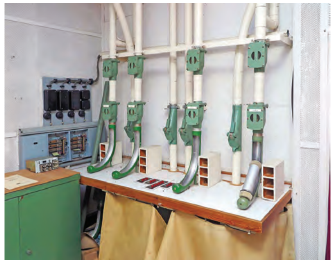
Pneumatic tubes enabled secure transfer of papers between rooms of Harnekop. Photo Clive Penfold
